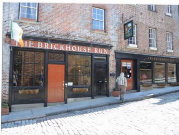
The Brickhouse Run Pub in Old Towne Petersburg
