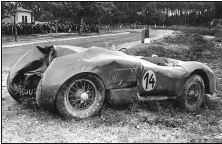
Duncan's Jaguar meets Portuguese power-pole pole
