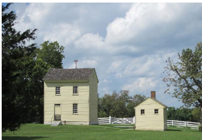
Water Reservoir Building at Shaker Village. Note "fill" flag on roof.
