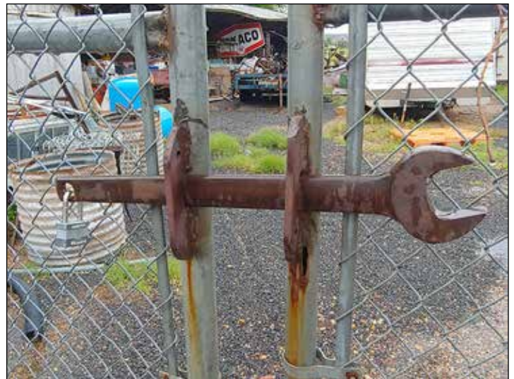
David Harrison submitted this crude, yet elegant, gate lock crafted from a large open-ended wrench and other bits and pieces laying about.
