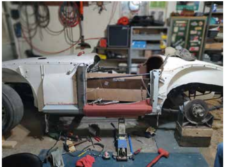
New doorsills and B Posts are installed.
